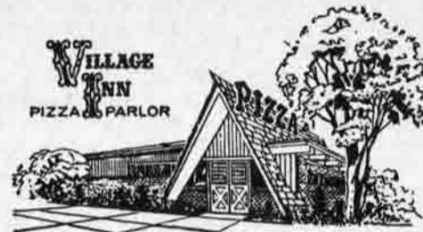
Natural Bridge One Block East of Brown Rd. Phone: 423-5300
